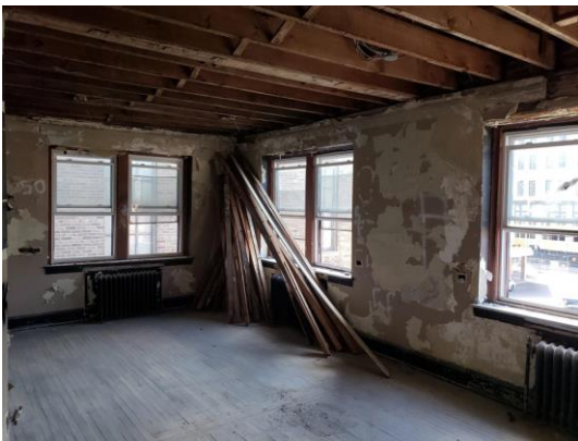
a studio being renovated at 219 East Hanover Street
